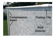
You need to leave a 1" gap between lengths of coping. Each coping gap should be offset from a wall joint by at least 2-3 feet. Once
