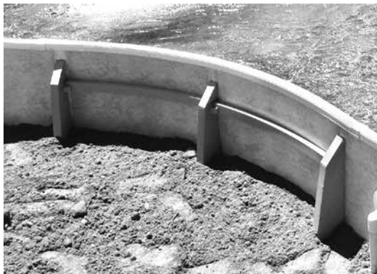
Semi-Inground with Structural Bracing
