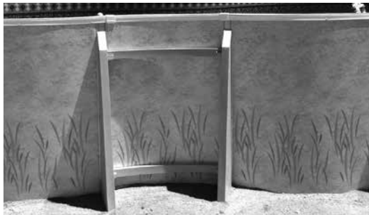
Aboveground with Structural Bracing
