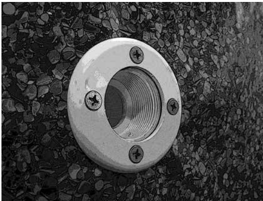
Return faceplate installed.
