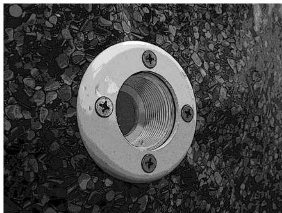
Return faceplate installed.
