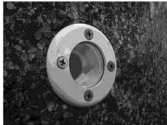
Return faceplate installed.
