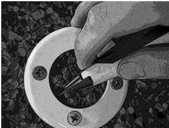
Trim liner from return opening.
