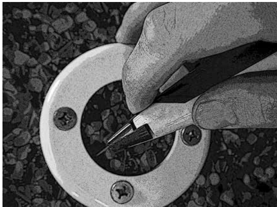
Trim liner from return opening.
