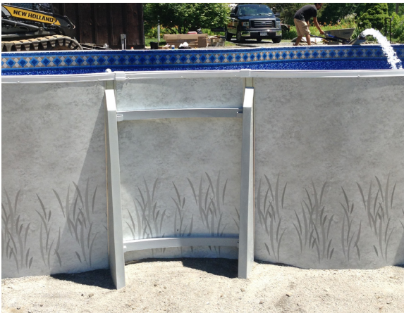
Aboveground Freeform with Structural Bracing installed.
