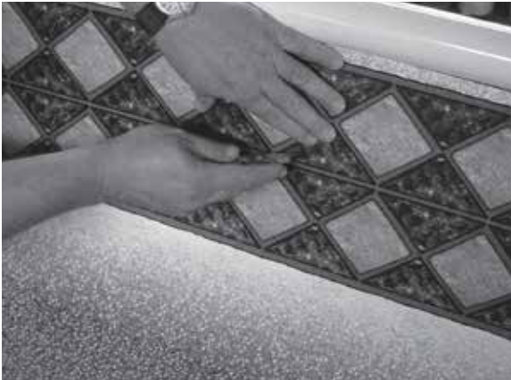
Locate screw holes for faceplate.
