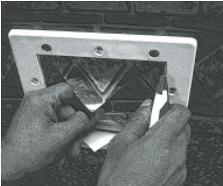
Trim liner from skimmer opening.
