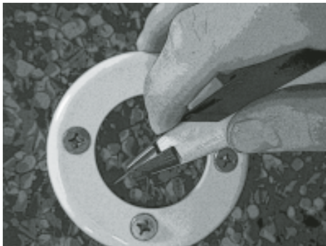
Trim liner from return opening.
