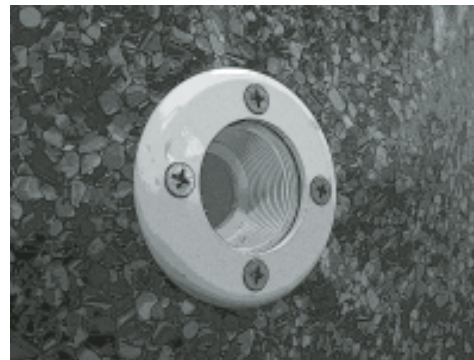
Return faceplate installed.
